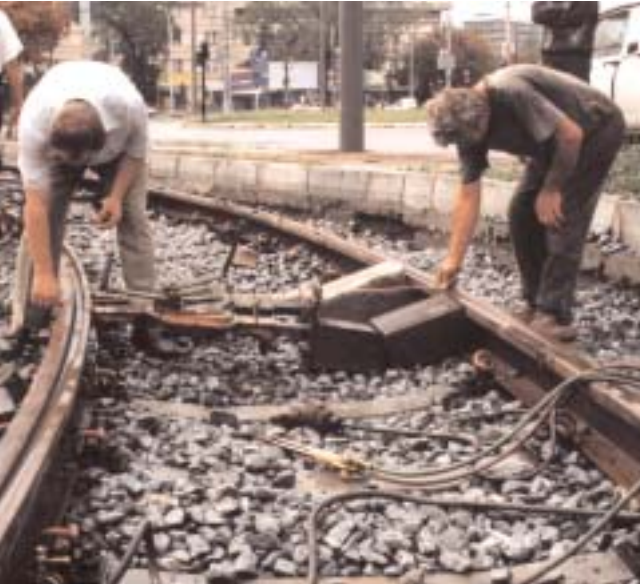
Figure 2. Alignment of the rail, an important task.
