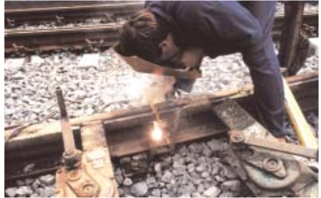
Figure 4. Welding of the rail foot.
