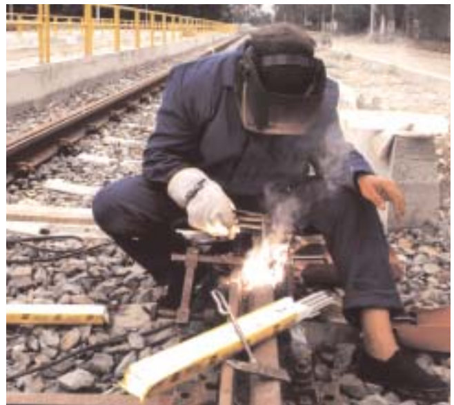
Figure 5. Mould welding with OK 74.78. Note the use of electrodes from VacPac vacuum packaging.
