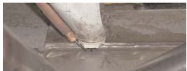
Figure 2. SCW™ set up showing the leading position of the cold wire to the left of the wire electrode (welding direction is to the left).
