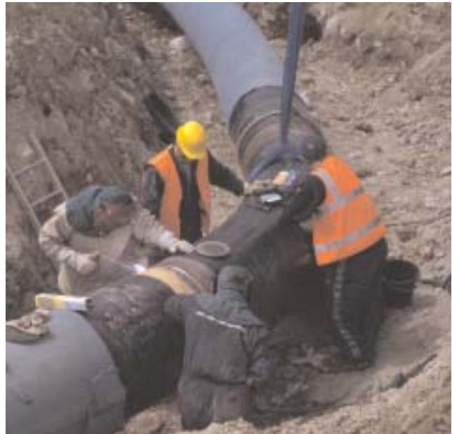
Figure 5. Downhill welding of a tie-in with Pipeweld 6010 cellulosic electrodes.
