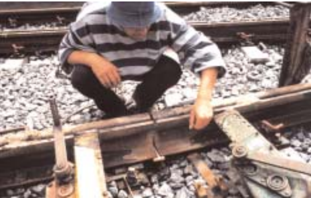
Figure 3. Placement of the ceramic backing strip OK Backing 21.21.
