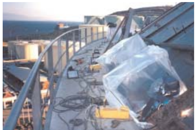
Figure 4. One of the LNG tanks for Egegaz under construction.
